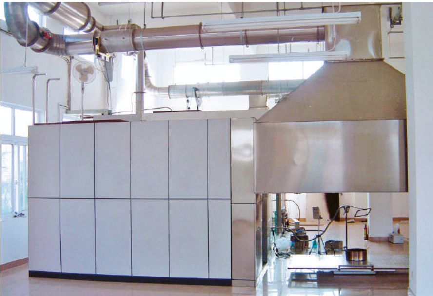
On-site system in a fire research institute
